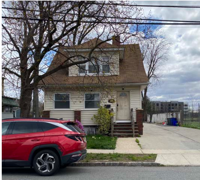
Photo 4: 35 Lawrence Street is a single-family dwelling with a building height of 2 stories.
