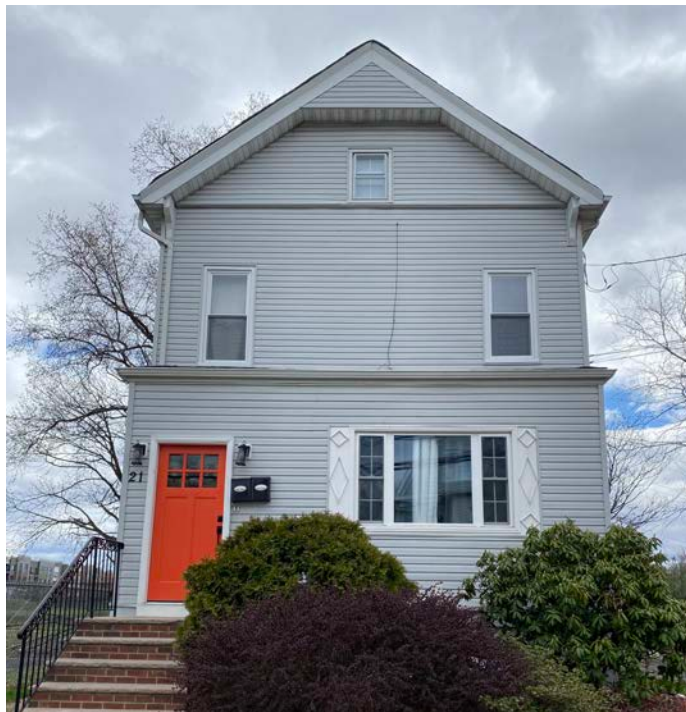
Photos 5: 21 Lawrence Street is a two-family dwelling with a building height of 2.5 stories.
